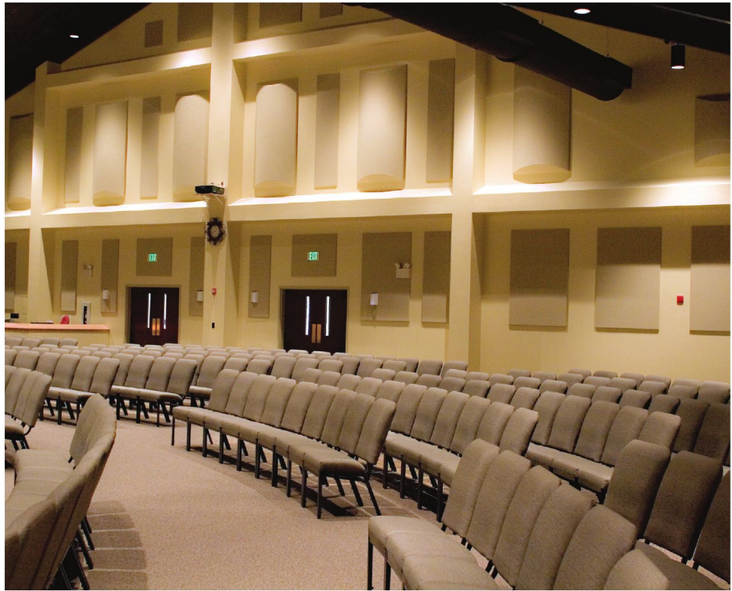
This church, located in Chester, Virginia, uses fiberglass absorbers around the room to lower the overall intensity of the sound and cut down the specular reflections from the large amount of wall space. They also added large barrel diffusers, which not only further break up the specular reflections, but function as bass traps due to their large resonant cavity filled with fiberglass batting.
