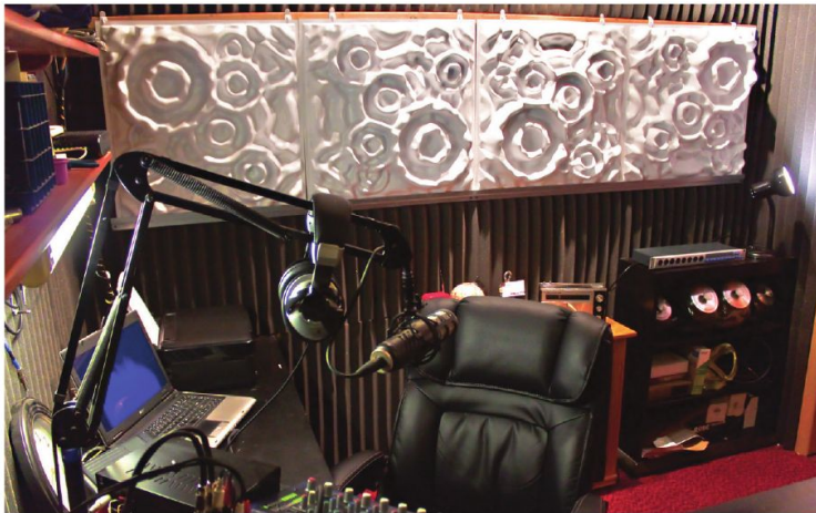
This smaller broadcast studio (88.7 WBWV–Beckley, West Virginia) uses a room completely covered in acoustic wedge foam, with diffusers placed to the rear at ear-level to spread some of the energy around the room—and keep it from sounding claustrophobic.
