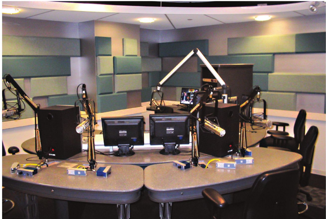
Similar environments (above and on page 26) may use different methods to achieve the desired acoustic outcome. This large broadcast studio (iHeart NY, formerly ClearChannel) uses an array of absorbent fiberglass panels spaced around the room and an irregular ceiling design to tame the acoustics of the room.
